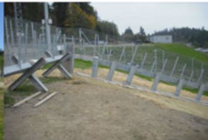
Perimeter Intrusion Detection and Assessment System (PIDAS) SWFLANT
